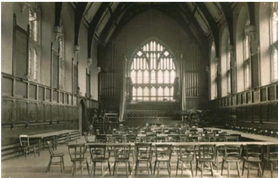
The interior of the Big School, Clifton College, in the 1920s.
