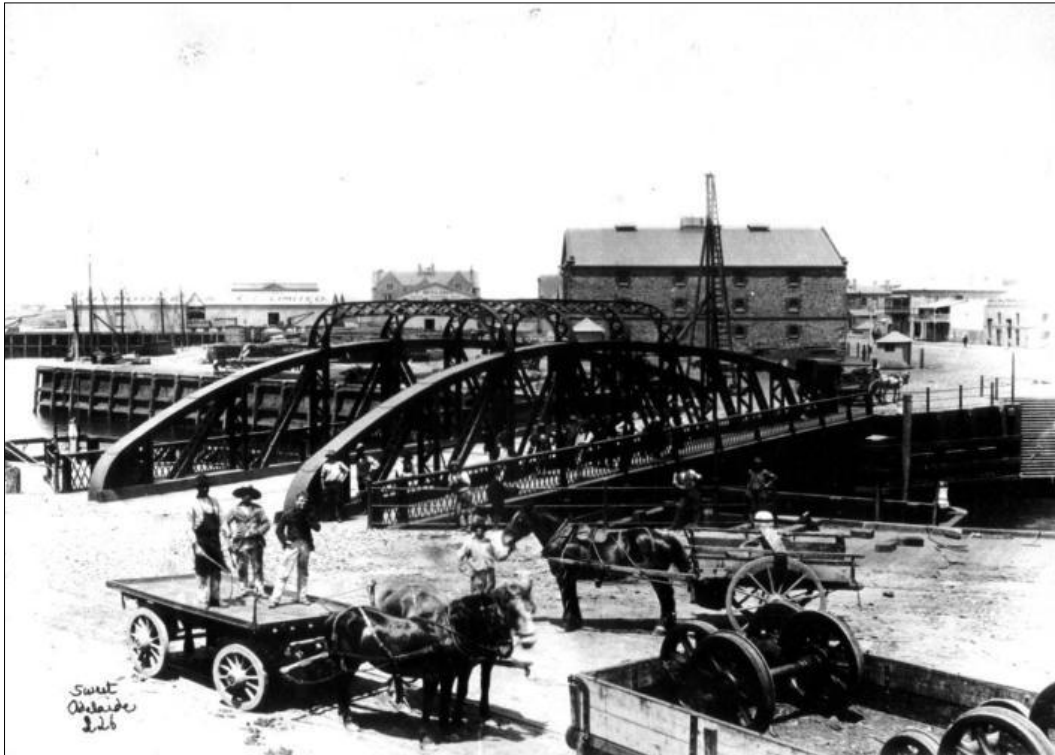
Adelaide's 19th Century bridges.
