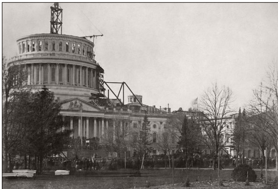
The Capitol, Washington, under construction.
