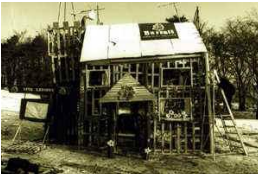
Tim Hunkin's pyrotechnic house under construction.
