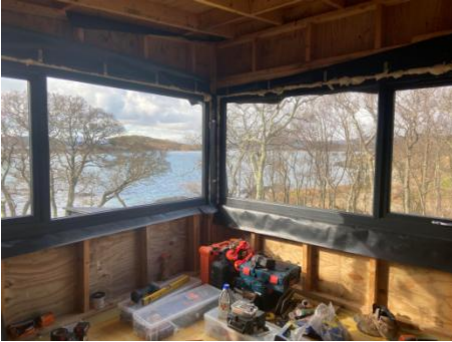
The bothy under construction.
