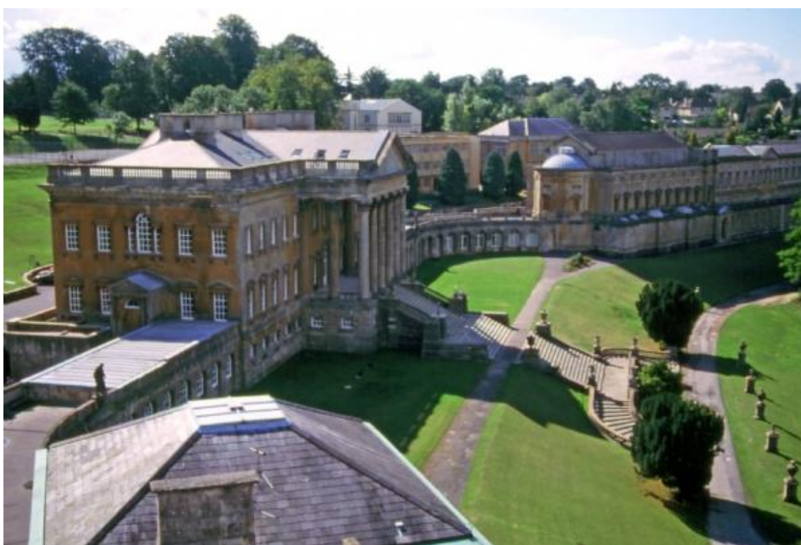
Prior Park College, with its elegant Georgian buildings overlooking Bath
