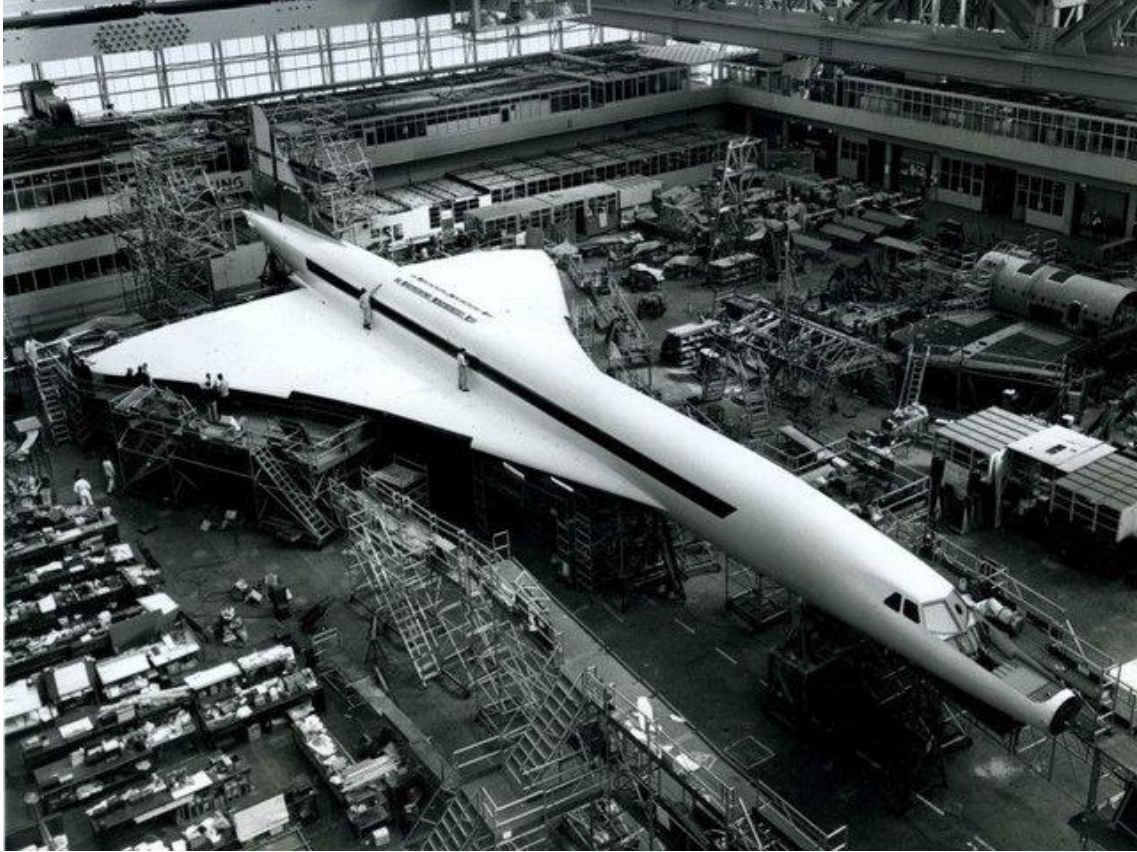
Prototype assembly at BAC Filton, 1970.
