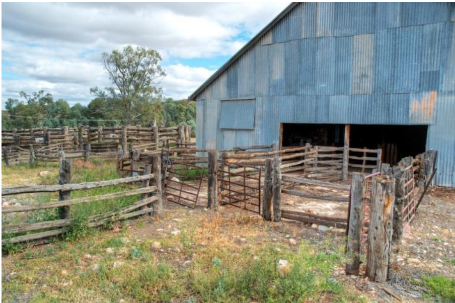
Wool shed and yards at Balcanoona sheep station.
