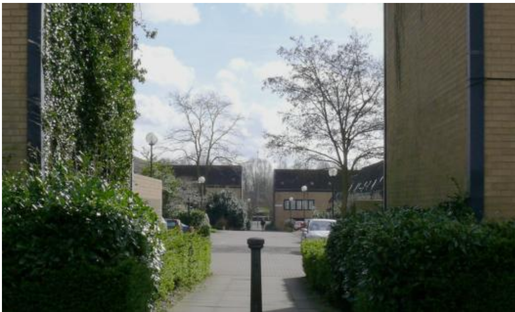
Housing scheme in Central Milton Keys by Spence + Webster.
