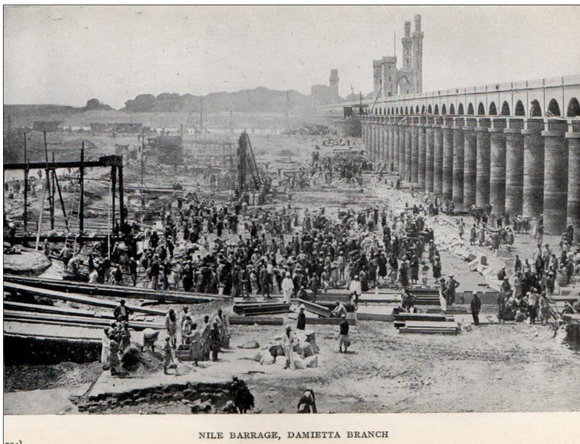
1890 Delta Barrage – Damietta Branch
