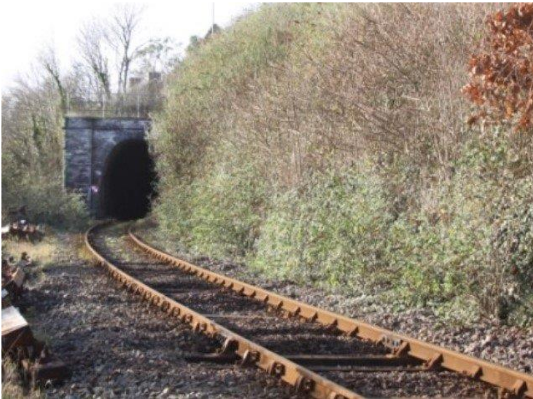
Railway Tunnel on the other side of Penhelig
