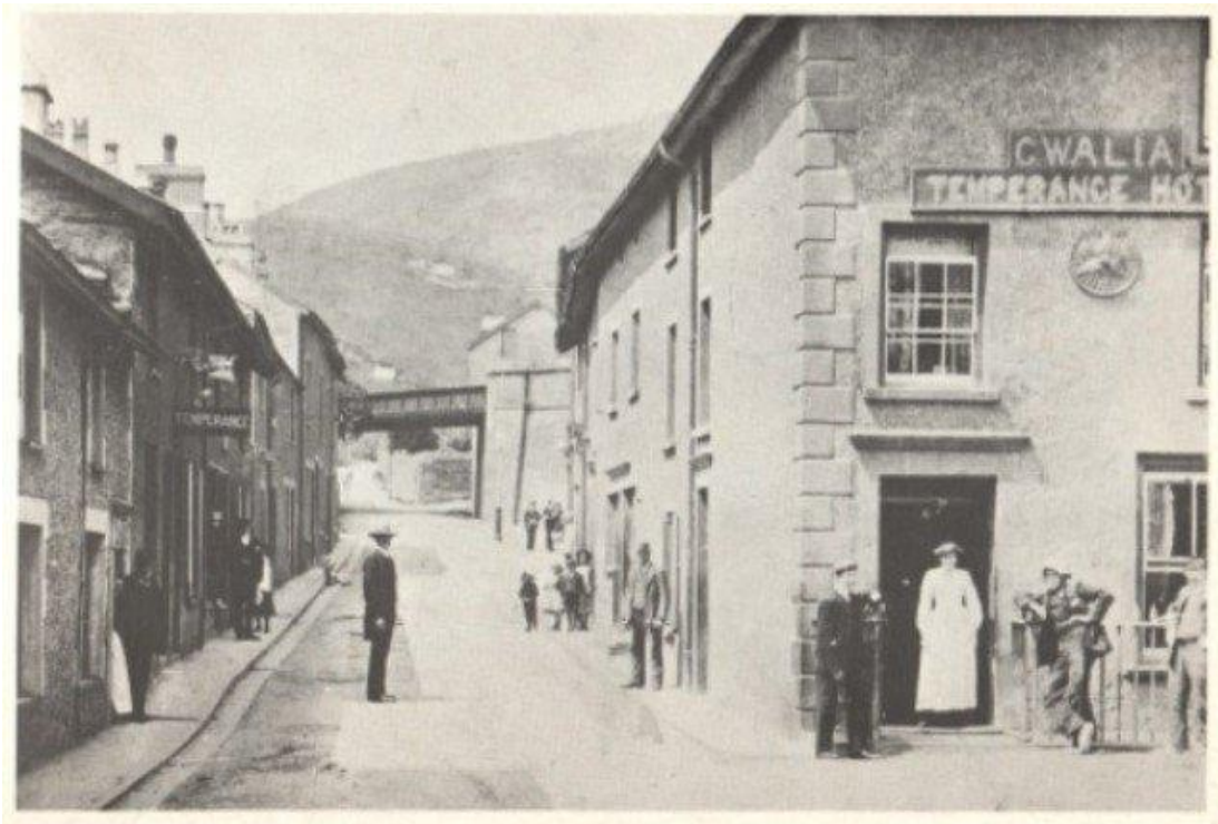
Photograph of the Temperance Hotel in Chapel Square, showing the bridge over Copper Hill Street in the background in 1867. Source: Hugh M. Lewis. Pages of Time.
