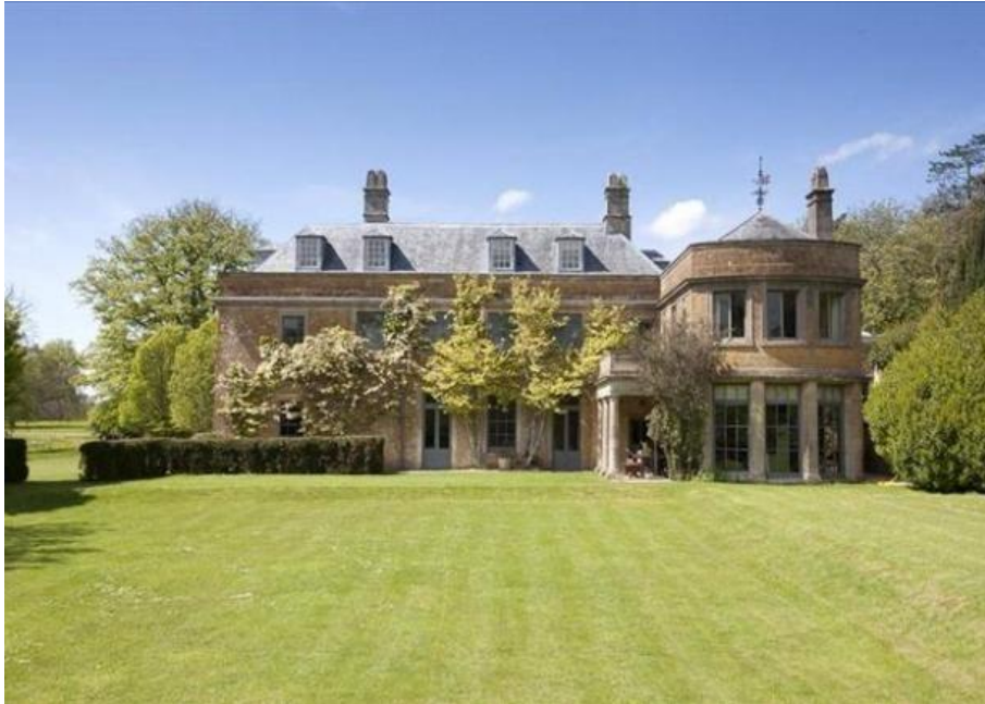
Hadspen House, now a hotel.
