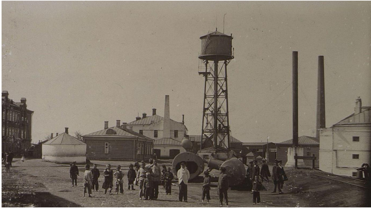
Courtyard of the Rabeneck factory at Shchelkovo, early 20C
