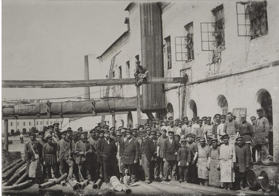
Workers at the Ludwig Rabeneck factory during heating improvements, about 1890
