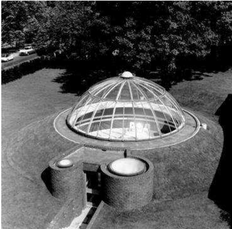
The underground pool at the Schreiber House
