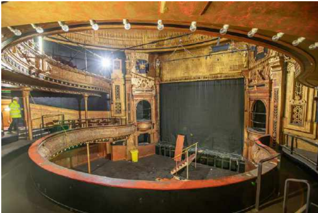
Citizen's Theatre interior during a recent refurbishment
