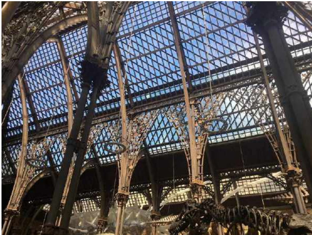
The exuberant wrought iron structure of the Oxford Natural History Museum's roof.
