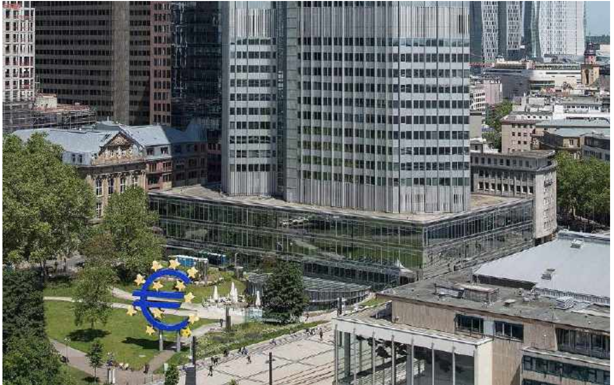
Salomon took the upper floor of the plinth in the Eurotower, providing very large open floor space. The Frankfurt New Opera house in the foreground.
