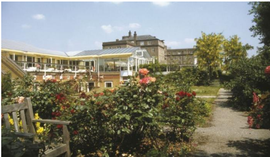
Lambeth Community Care Centre, completed, in mature garden.
