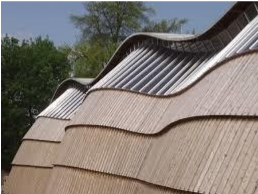
The roof of the gridshell building at the Weald and Downland Museum.
