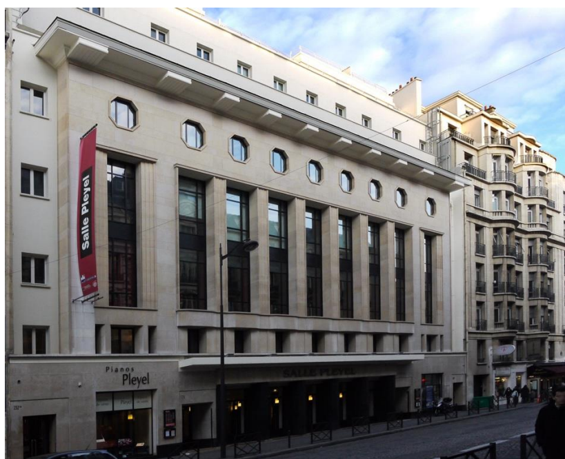
Salle Pleyel, opened in 1927, designed by acoustician Gustave Lyon together with architect Jacques Marcel Auburtin
