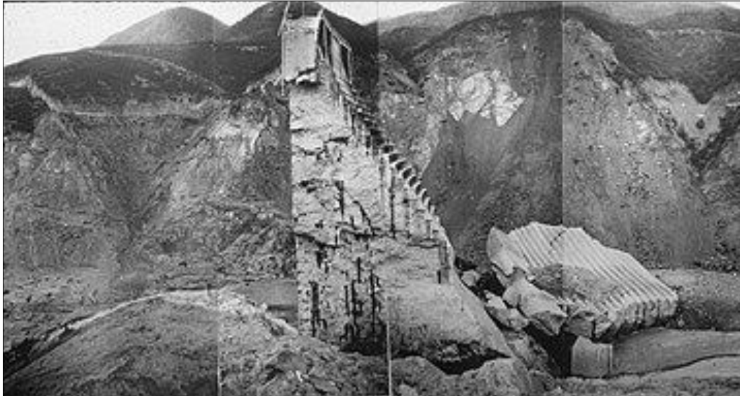
Cross section of St. Francis Dam after collapse.
