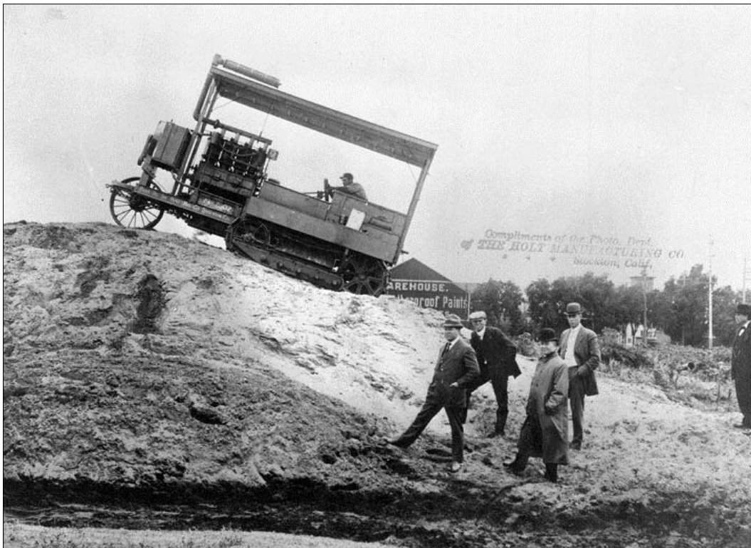
The first caterpillar tractors ever built were used in 1907 on the Elizabeth Lake tunnel.
