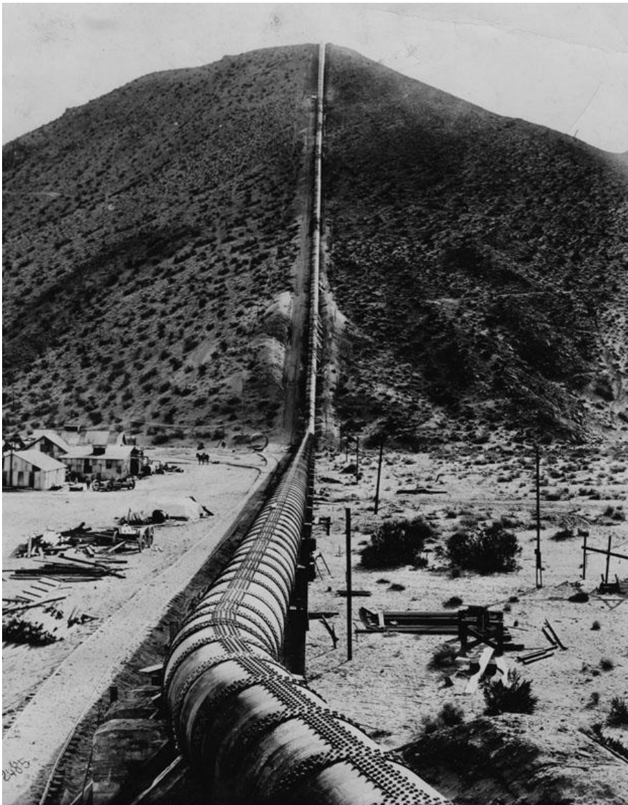
The Jawbone Siphon almost completed in 1913.
