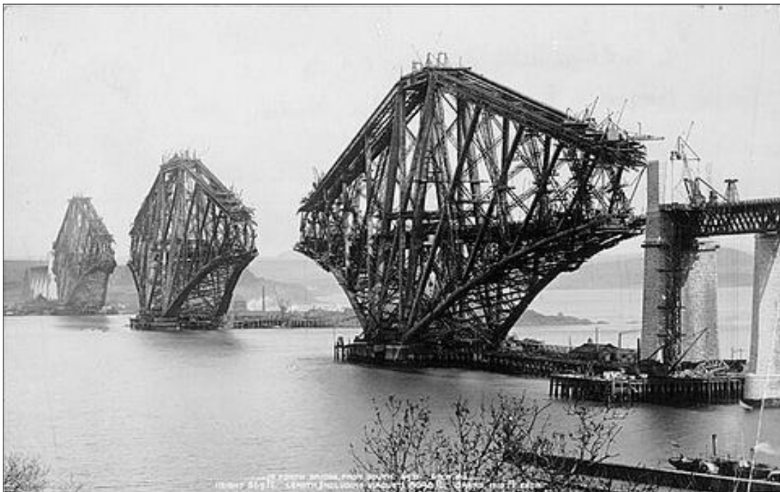
Forth Railway Bridge under construction in the 1880s.
