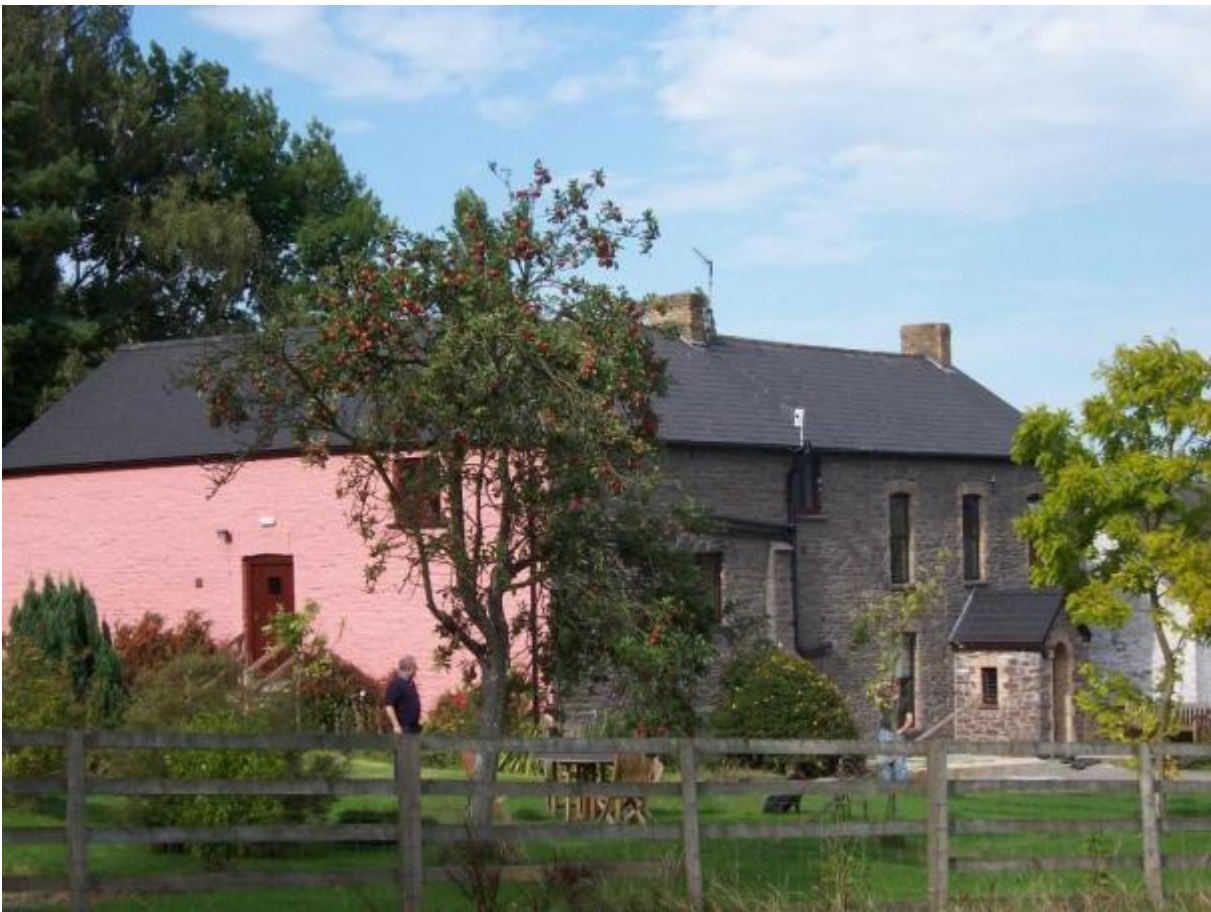
Brynderwen, at Llangorse, near Abergavenny, which was bought by the Luckocks in 1912. They overhauled the drains and put in electric light.
