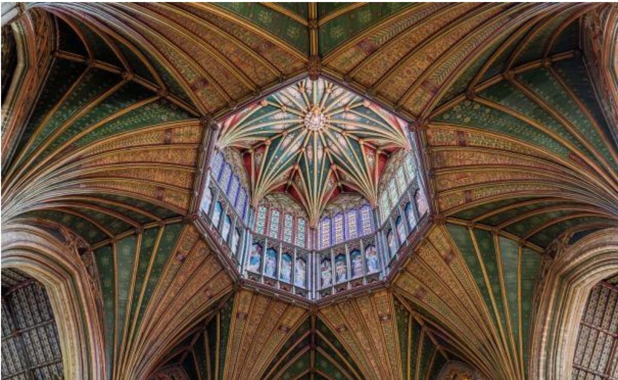
Interior view of the transept lantern at Ely Cathedral.
