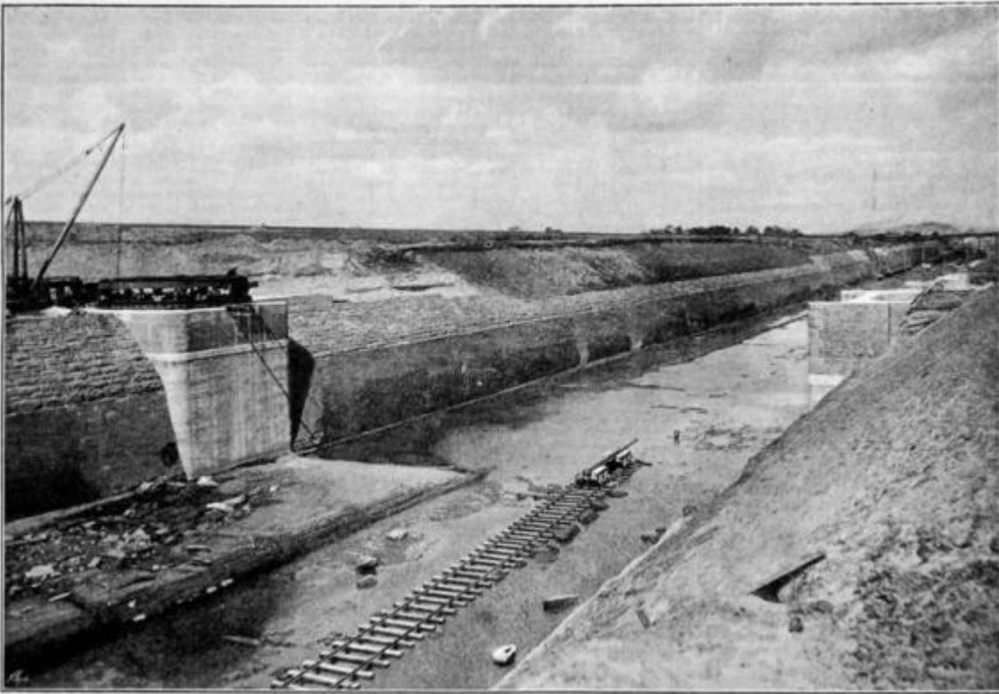
FIG. 7. SWING BRIDGE AT MOORLANE, NEAR WARRINGTON.
