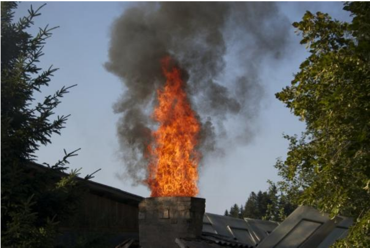
A chimney fire is the combustion of residue deposits of soot or creosote, on the inner surfaces of the chimney.
