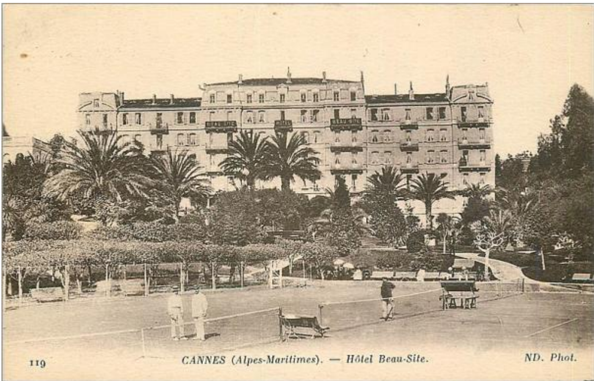
Hotel Beau Site, Cannes, where the Luckock family stayed in 1911. The Riviera Tennis Tournament was held on the courts of the hotel.
