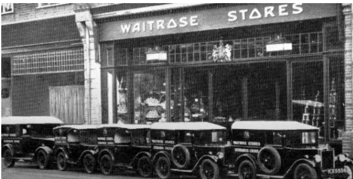
Original Waitrose shop in Gerrards Cross.
