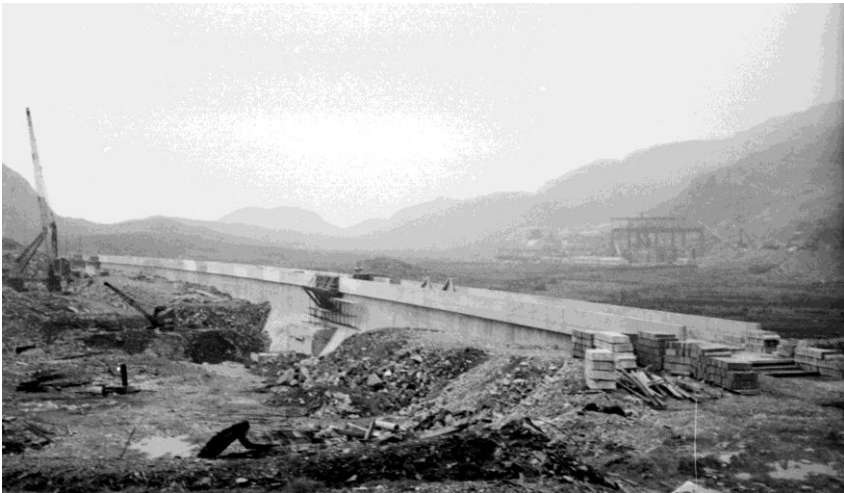
March 1960, Tanygrisiau pump storage scheme - the dam and powerhouse take shape
