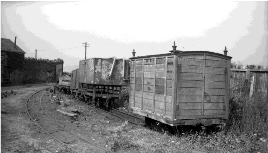
August 1955, Boston Lodge. The 'hearse' on the old inspection pit
