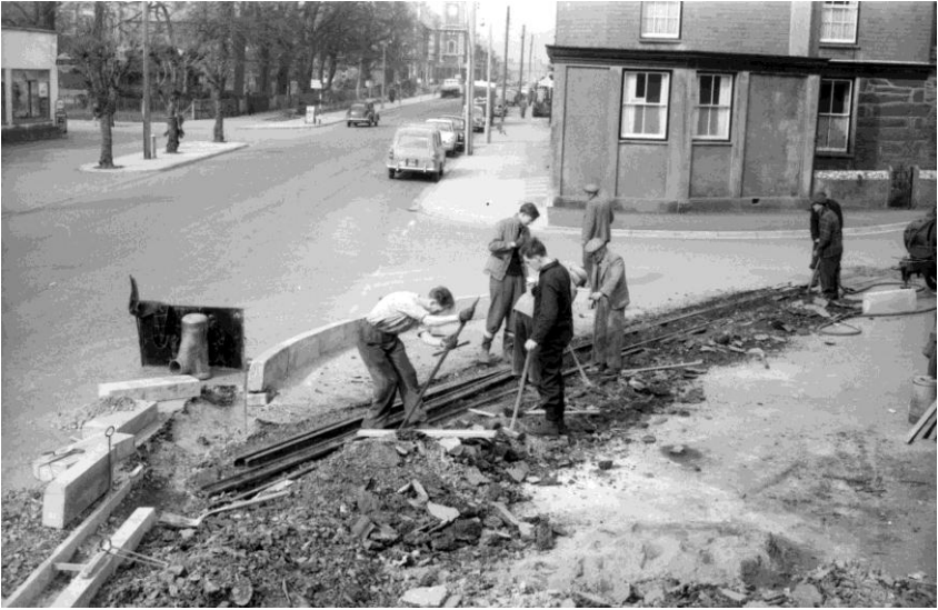
March 1960, the Cambridge University Platelayers lift the last of the Croesor tramway rails in Portmadoc High Street
