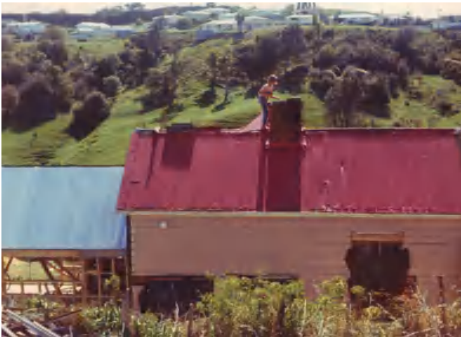
1974: JJ (Jeremy James) on the roof of the house at Shakespeare Road, Bastia Hill, Whanganui. Taking the chimney down brick by brick. No need for safety hats or scaffolding or ropes.
