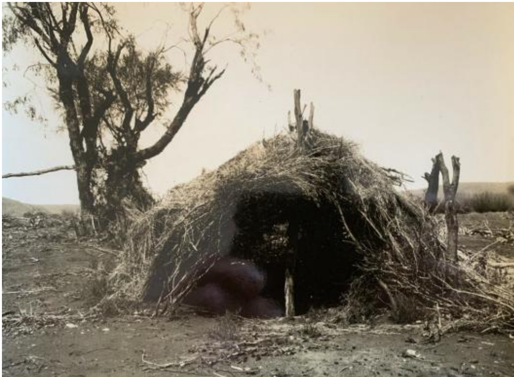
A gunyah is an Aboriginal bush hut, typically made of sheets of bark and branches.
