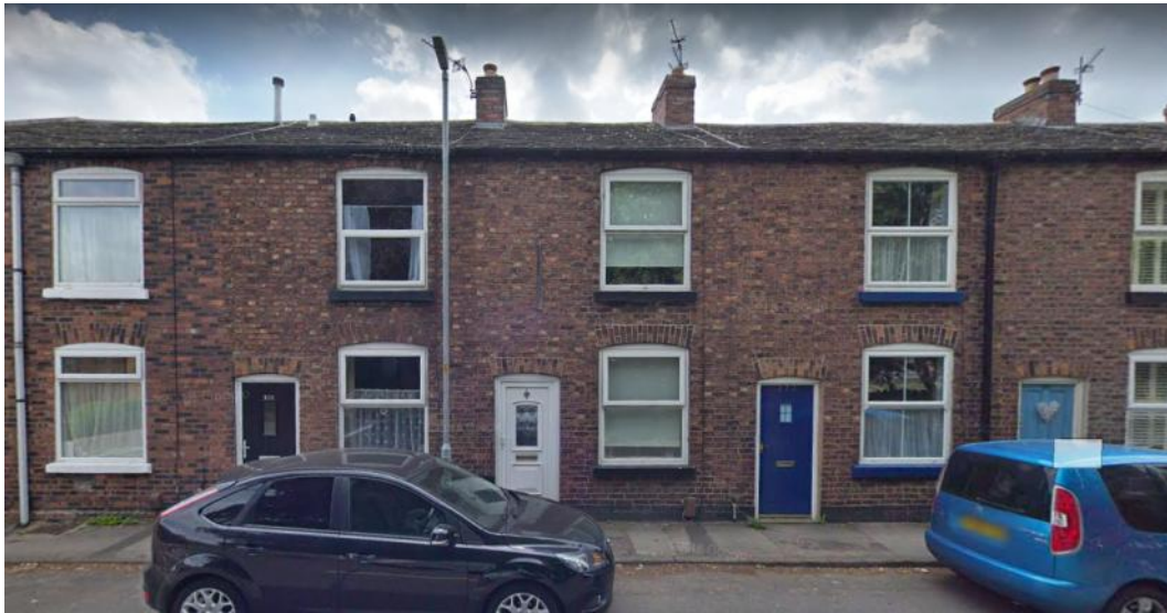
222 Black Road in 2021. It is the house with the dark blue front door and window sills.
