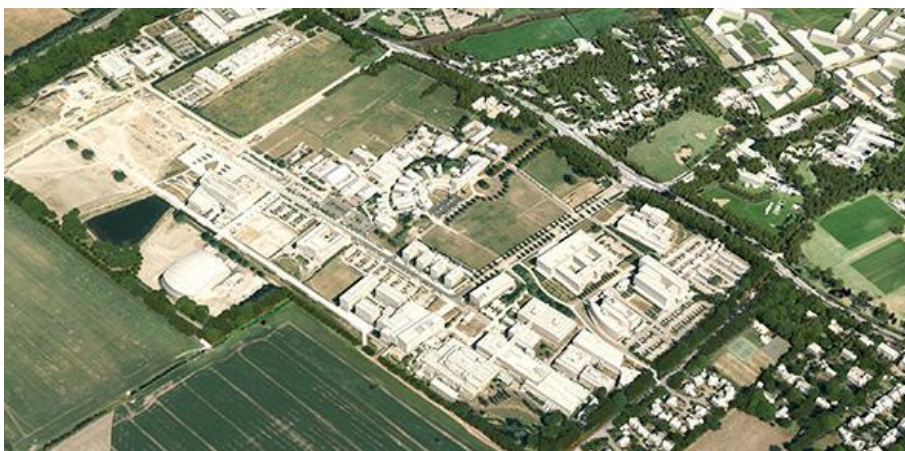
The West Cambridge Site. Cavendish II occupies the bottom corner.
