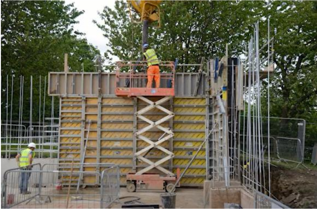
Pouring into the formwork.
