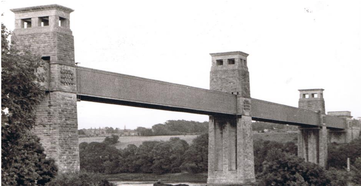
Illus. 7.3: The Britannia Bridge as it was in 1962. 31
