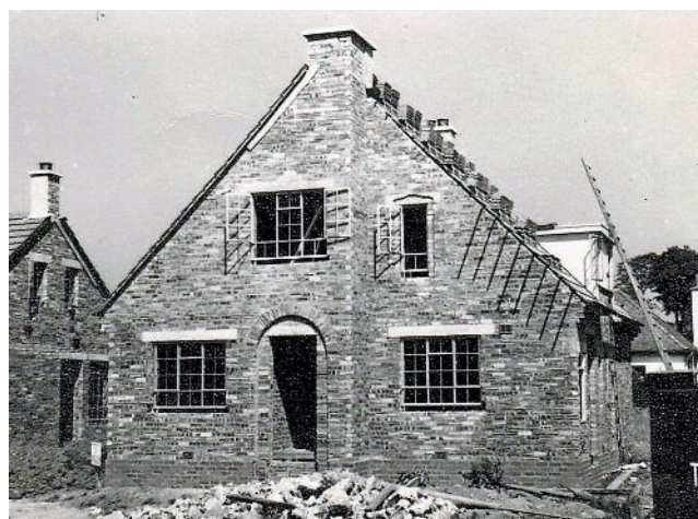
13 Sinclair Ave, Bearsden, our new house being built, 1957
