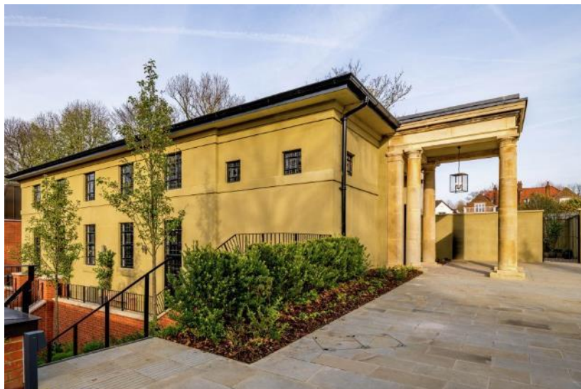
The former Westfield College Chapel – now a domestic residence
