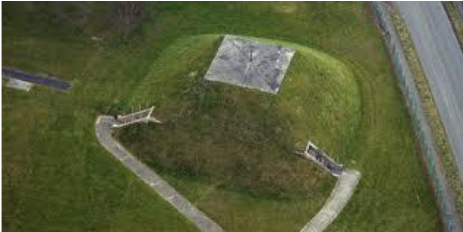
An entrance to the Corsham tunnels.
