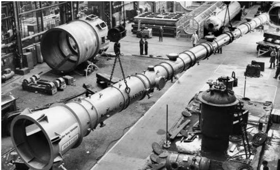
A fractionating tower under construction.
