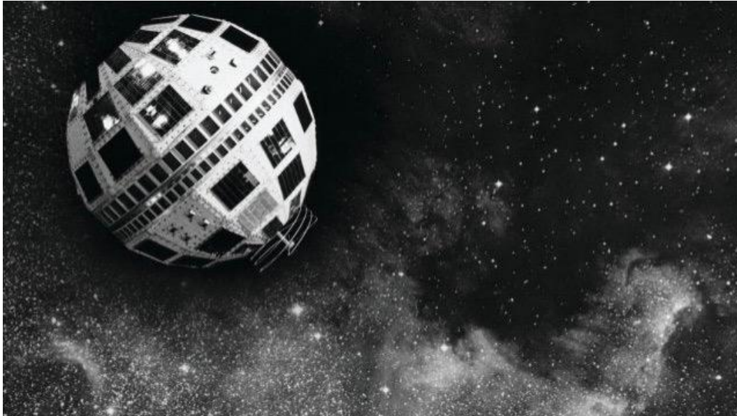
Telstar 1, built by Bell Laboratories and launched in 1962.
