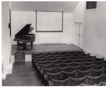
Stable converted to small hall.
