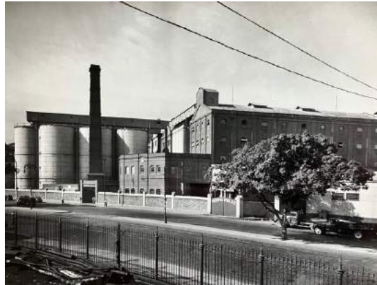
Rio mill and silos in the port area
