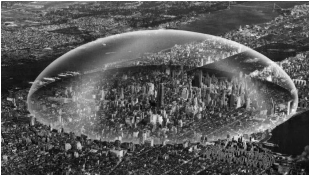
Visualisation of Buckminster Fuller's proposed dome over Manhattan. It was intended to keep out the rain and modify the climate to reduce energy consumption of buildings.
