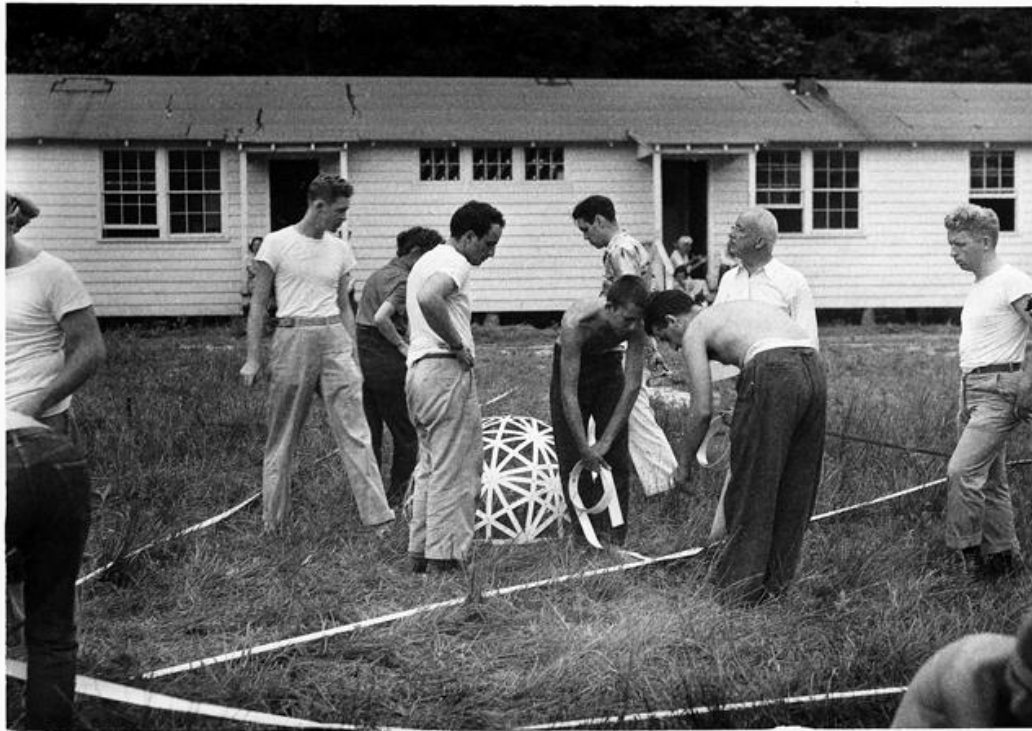
Bucky works with students on the construction of the Supine Dome at Black Mountain College in North Carolina in 1948. Courtesy Winslow Wedin/The Estate of R. Buckminster Fuller.
