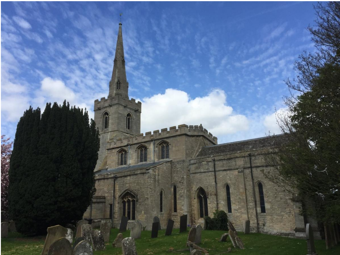
St Mary, Wilsford, 11-15C, in Ancaster limestone. Restored 1860 by Kirk and Parry of Sleaford, then one of the largest British design and contracting firms, made rich by railway construction.
