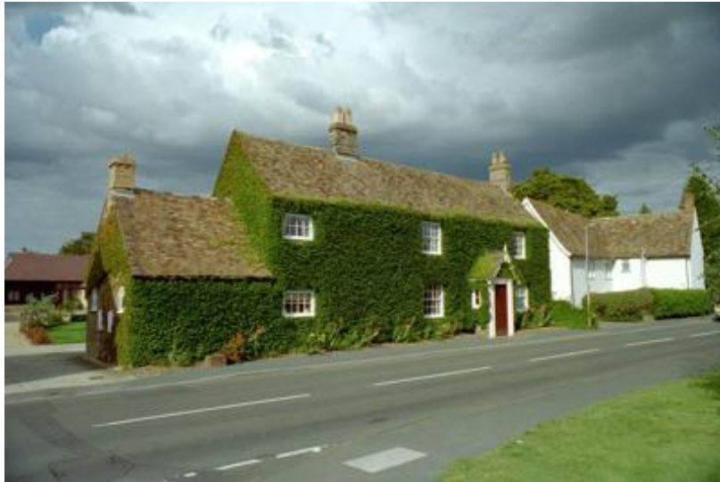
Low Farm, Buckden, Cambridgeshire. Grade II listed early 19C farmhouse.
