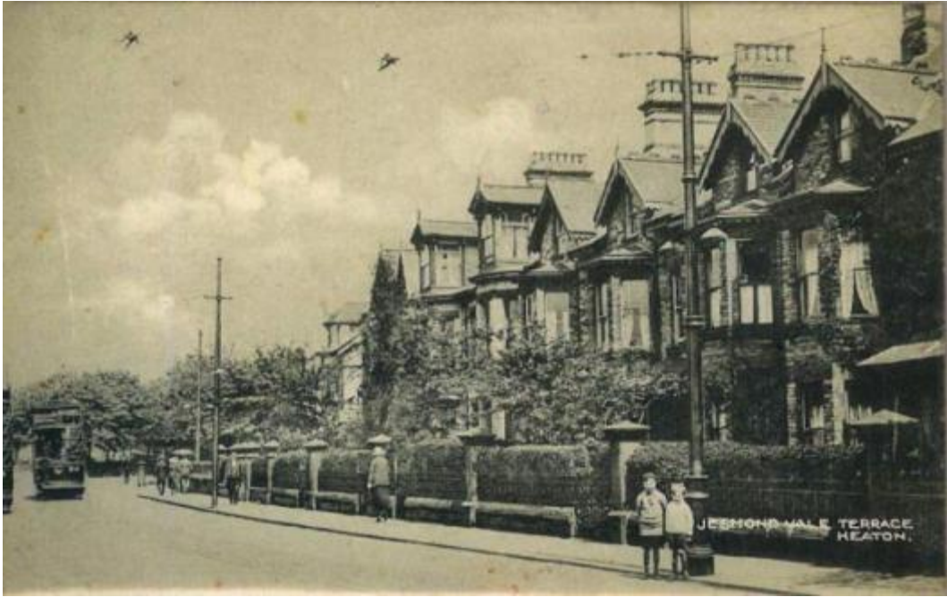
Jesmond Vale Terrace, Heaton.
