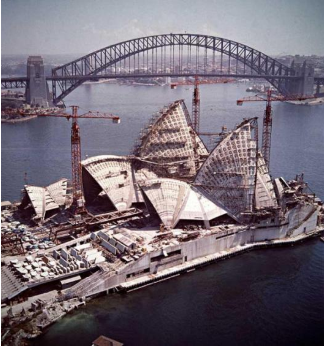
Sydney Opera House under construction - 5 shells erected.
