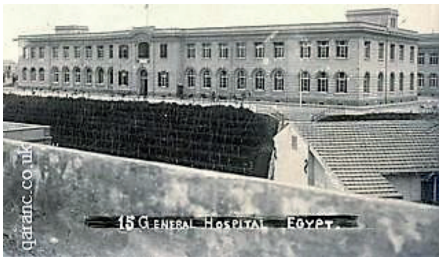
No. 15 General Hospital, Egypt.
